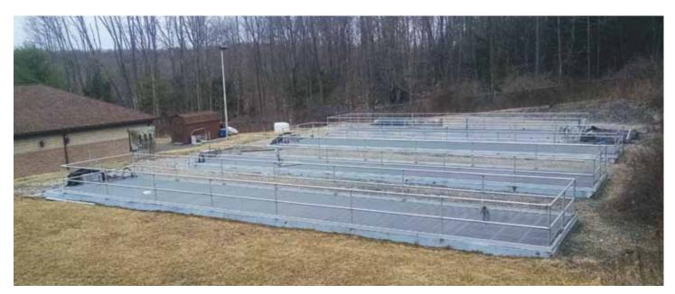
This facility was monitored for two years to evaluate compliance with the total nitrogen discharge limits set by the Chesapeake Bay Biological Nutrient Removal requirements. It met or exceeded those limits without any chemical addition. The BNJSA saved over \$1 million by not having to construct clarifiers and related equipment.
