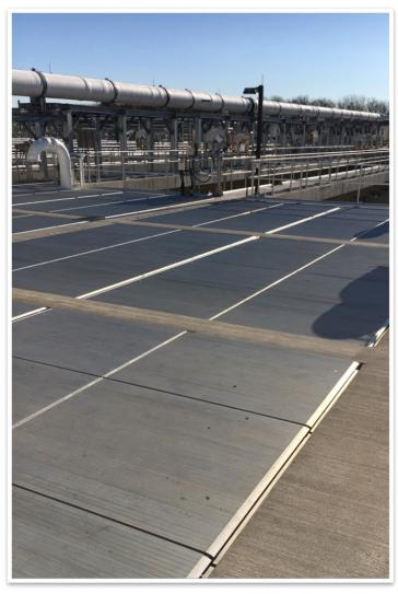
access to weirs, basins, blowers and other equipment located below the covers. This provides odor control and a safe working environment for plant operators. PMWI aluminum covers require little to no lifetime maintenance, reducing plant preservation costs and saves energy. Our covers are durable and strong enough to handle large loading requirements, allowing for safe navigation throughout the plant.
