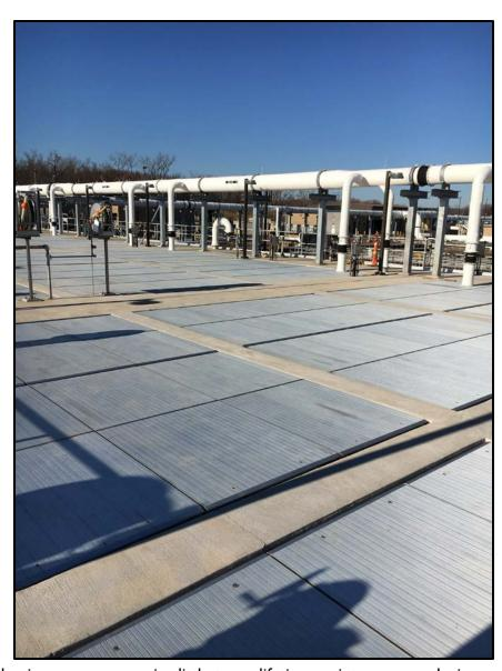
environment for plant operators. PMWI aluminum covers require little to no lifetime maintenance, reducing plant preservation costs and saves energy. Our covers are durable and strong enough to handle large loading requirements, allowing for safe navigation throughout the plant.
