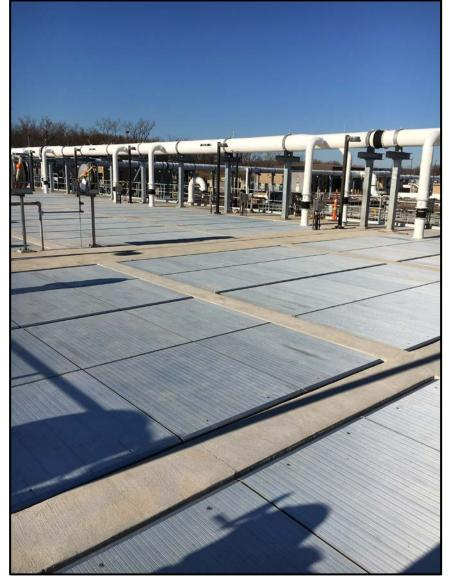
control and a safe working environment for plant operators. PMWI aluminum covers require little to no lifetime maintenance, reducing plant preservation costs and saves energy. Our covers are durable and strong enough to handle large loading requirements, allowing for safe navigation throughout the plant.
