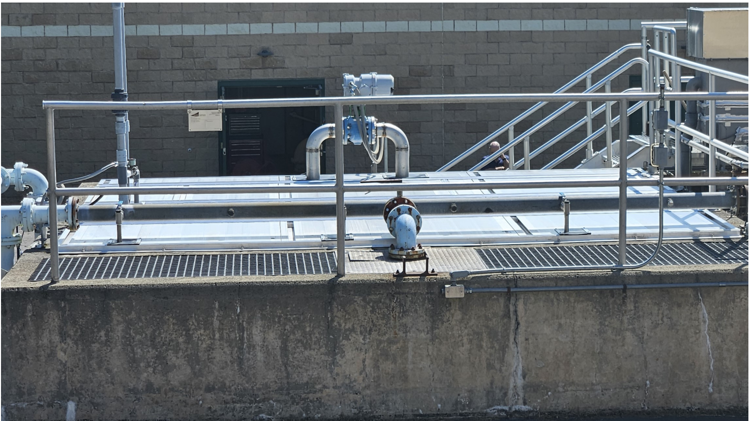
STANDARD-DUTY ALUMINUM INTERLOCKING FLAT PANEL COVERS (3 HINGED COVER PANELS SHOWN)
