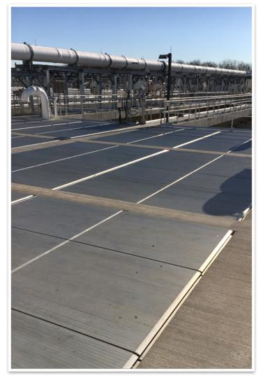
access to weirs, basins, blowers and other equipment located below the covers. This provides odor control and a safe working environment for plant operators. PMWI aluminum covers require little to no lifetime maintenance, reducing plant preservation costs and saves energy. Our covers are durable and strong enough to handle large loading requirements, allowing for safe navigation throughout the plant.
