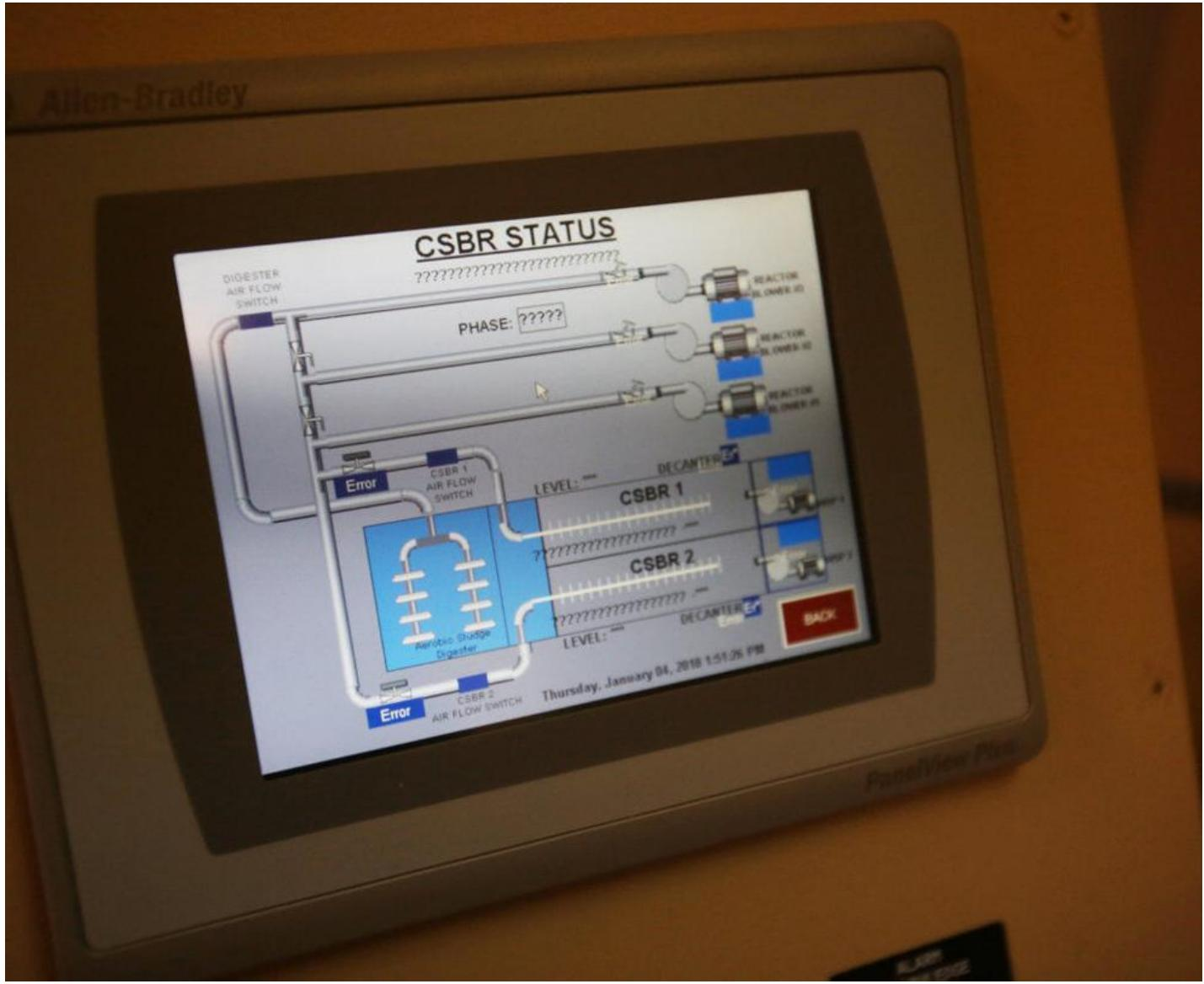
JAKE DANNA STEVENS / STAFF PHOTOGRAPHER Pleasant Mount Welding Inc. in Carbondale created a new control panel called the Human Machine Interface device. The panel is used to control a sequencing batch reactor.
